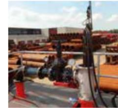
**4** The pump (with seal) is hung in the hoisting cable and inserted through the T-piece into the pipe.
