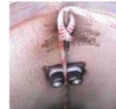
**5** Once the required depth is reached the hoisting cable is firmly anchored using cleats and the winch is removed.
