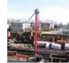
**3** The winch is bolted onto the T-piece top flange.
