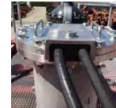
**6** The specially adapted cover, which incorporates the seal for the hydraulic hoses, is then bolted in place. The discharge hose is attached to the T-piece side connection.
