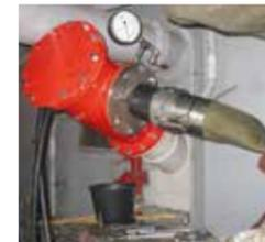
**8** After assuring the discharge hose is connected to the designated reception point, pumping can start.
